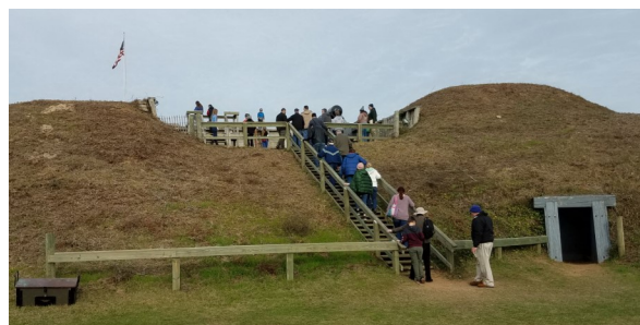
Visitors climb stairs to reach a traverse gun emplacement on Ft. Fisher's northern wall. Note the entrance to a bomb proof where defending troops would shelter or ammunition would be stored
